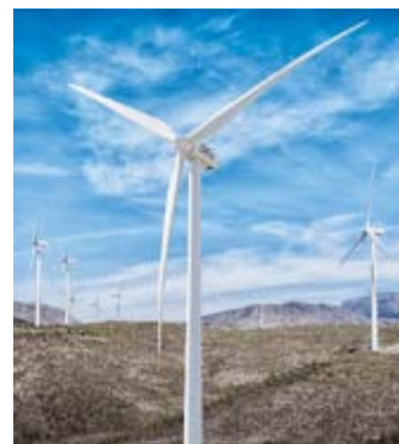
Throughout Central Queensland, there are several wind farms at different levels of progress. Picture: SUPPLIED
