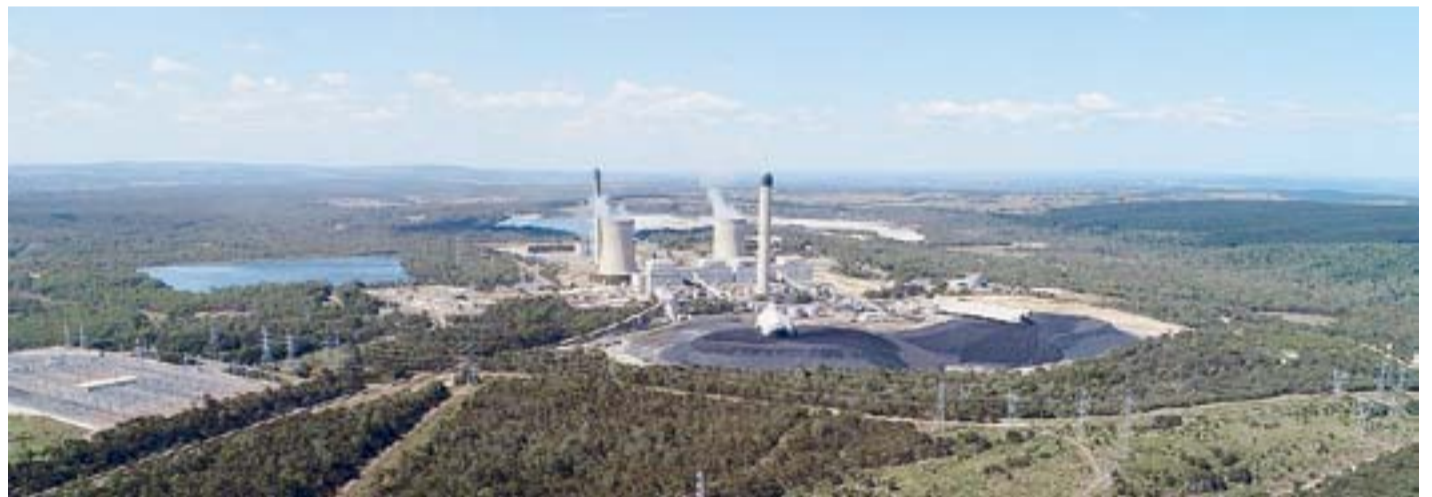
Stanwell is among the existing power stations set to share in $376 million for upgrades and maintenance in 2024-25. Picture: FILE
