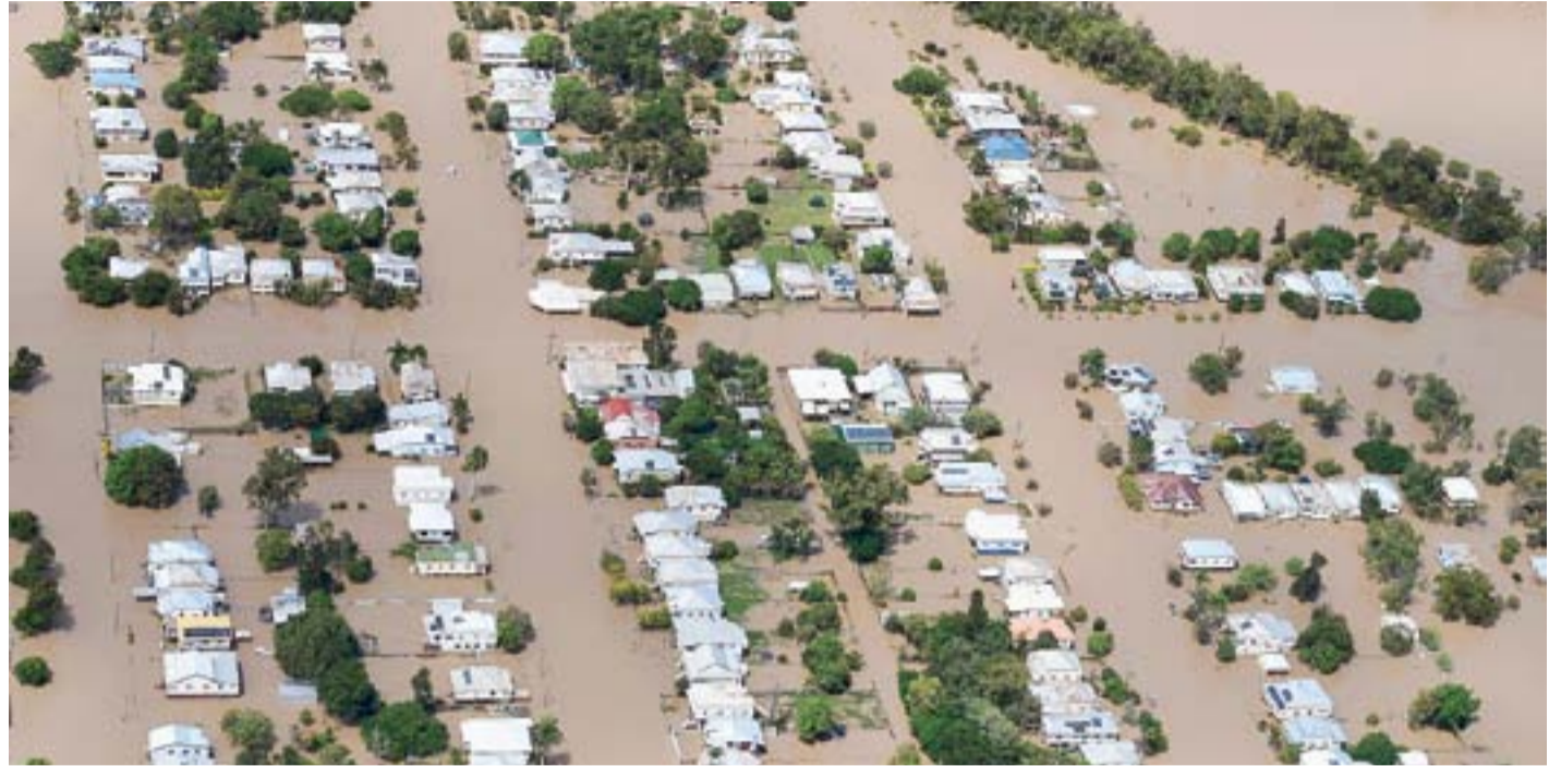
Houses are surrounded by floodwaters at Depot Hill on 6 April, 2017. Jason Foss says Central Queensland is not immune to natural disasters like floods, storms and fires. (AAP Image/Dan Peled)
