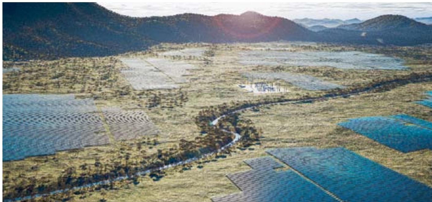
The $500 million Aldoga Solar Farm will feature up to 820,000 solar modules with the capacity to produce 480 megawatts at its peak.
