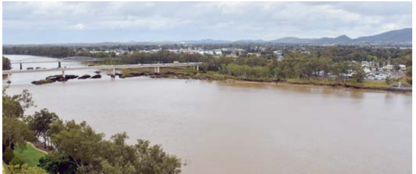
The establishment of a Marina Ferry Terminal and Facilities in the Fitzroy River is among the major projects touted by the Central Queensland Industry Collaborative.
