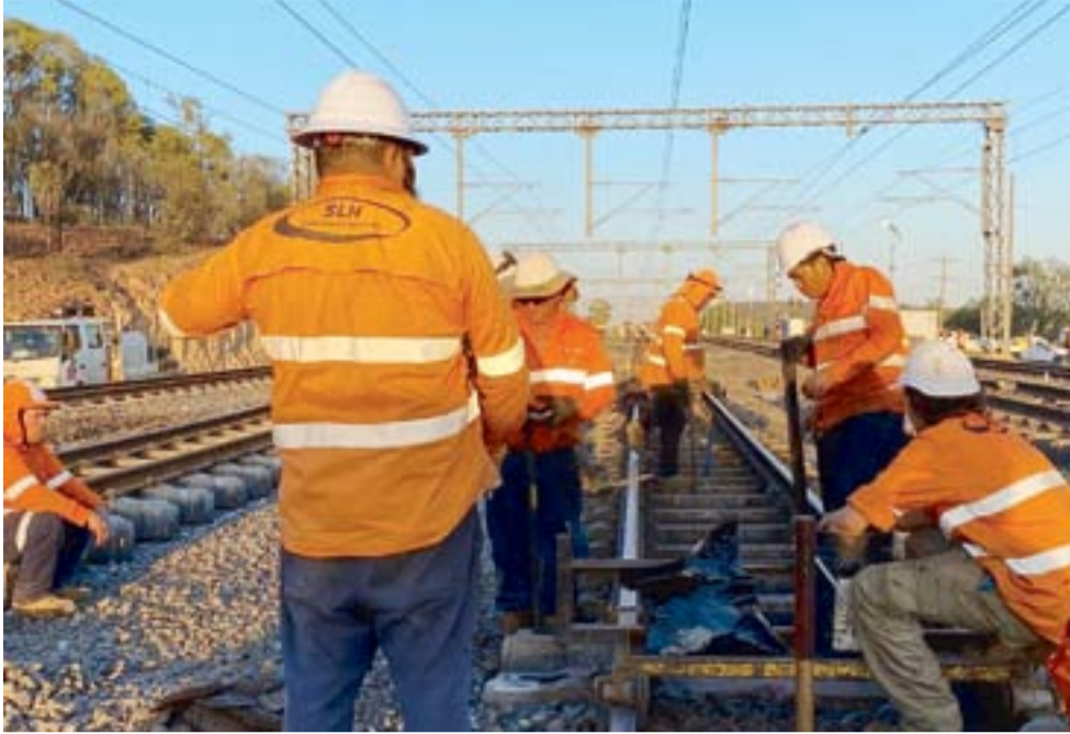
SLH crew with Rhomberg Crew Bluff Track Recon.
